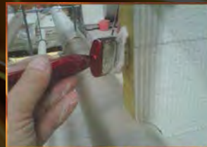
Buttering Up The Edges of The Intubatt
